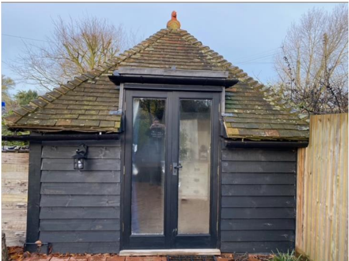
Figure 1: Existing annexe (entrance)
